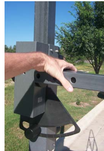
3. With pin removed, grasp mounting arm.
